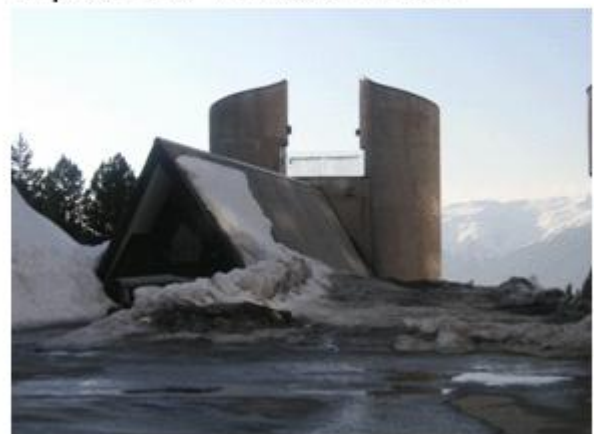
Top of Car Park Lift Exit
